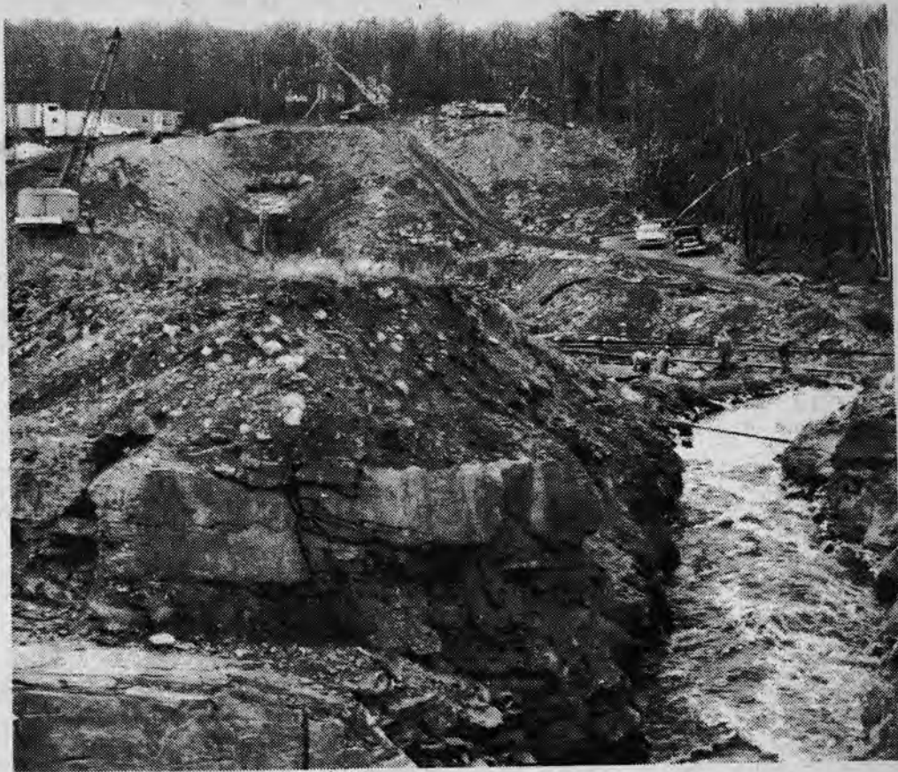
Tons of dirt and rock span across Shohola Creek, a few yards above Shohola Falls as construction workers change the flow of the creek in order to erect the monolithic concrete dam. The dam will be situated in the center area of the picture.
