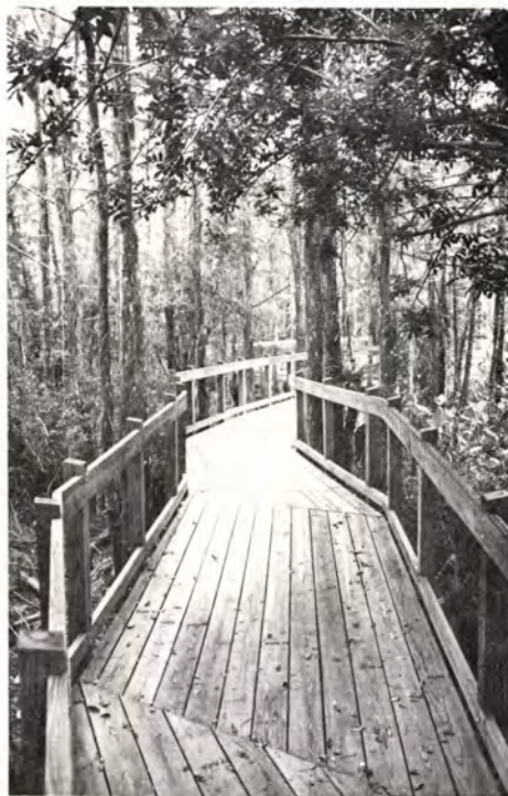
A boardwalk built by Project ABLE students, Ft. Myers, Florida.
