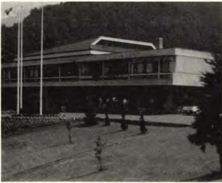
YMCA International Youth Center, Main building, office and dining room and meeting rooms, Japan.
